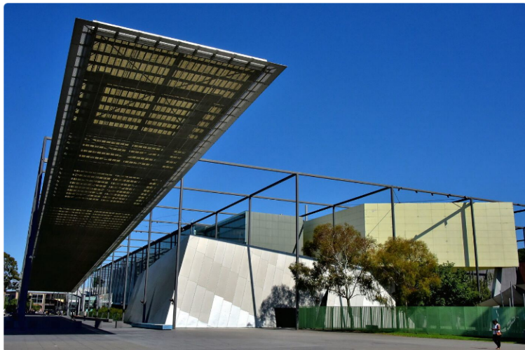
Melbourne Museum, eastern wing - adjacent to the site.
